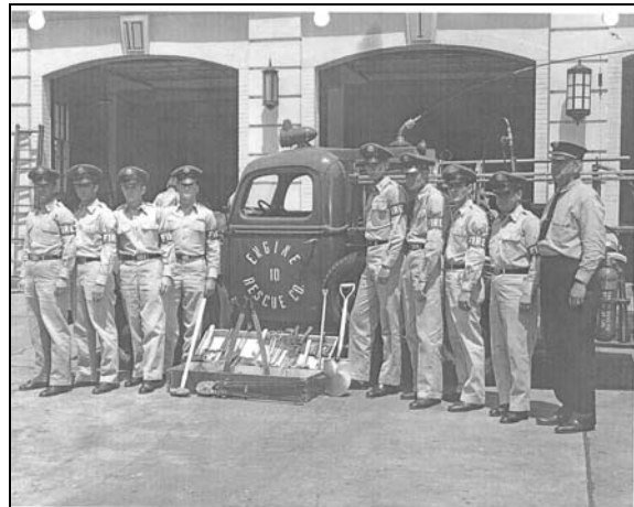
The first Air Force Aircraft Crash Rescue Truck, Engine 10, Rescue Company, MacDill AFB, Tampa, Florida, 1947-1959. Chief Frank Joseph built this unit on a half-ton Ford chassis. The elite rescue crew was credited with saving many aircraft crew members. Chief Lloyd W. Garner was crew chief of this specialized unit and received the Soldier's Medal, along with the rest of his crew, for rescuing a flight crew from a burning aircraft.
