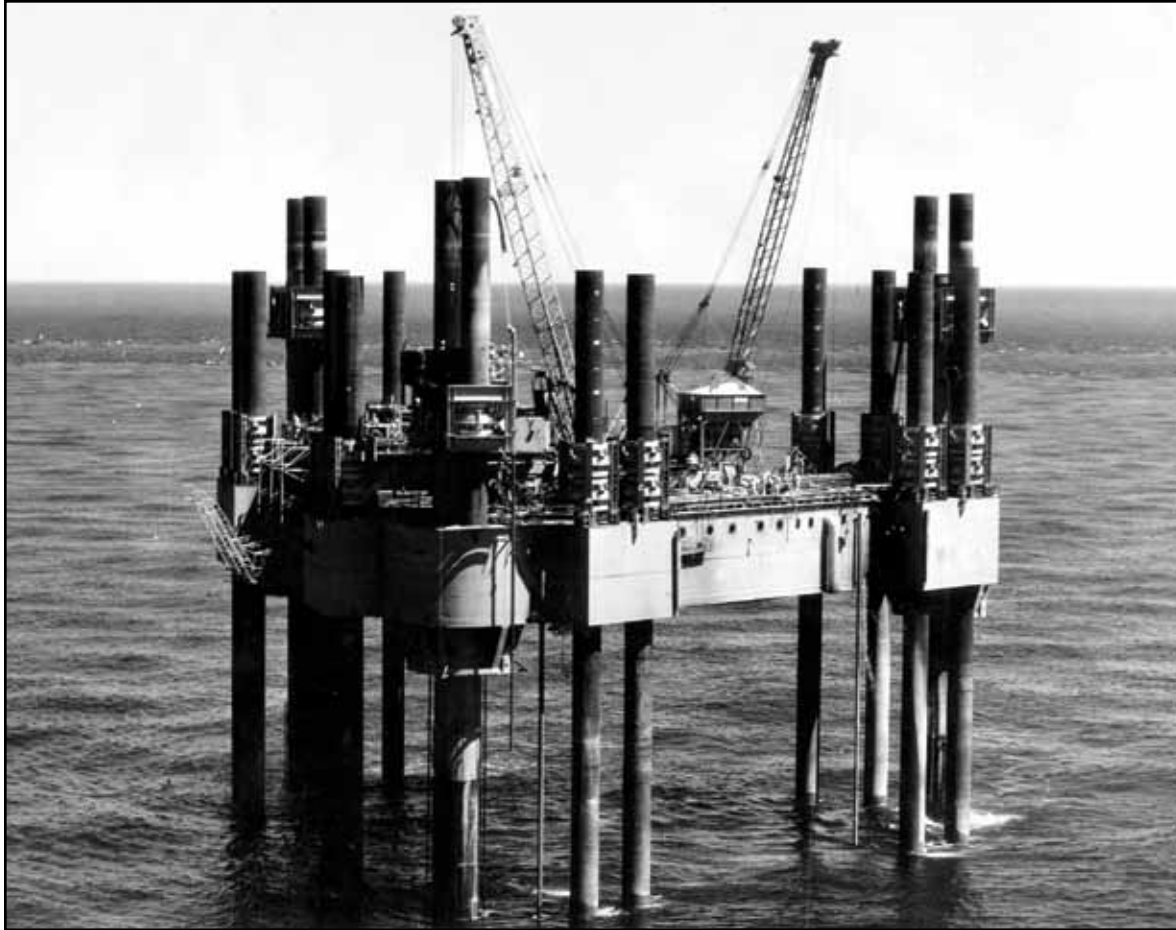
One of the Texas Tower sites under construction.
