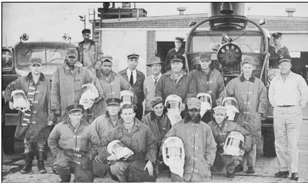
Members of the Tyndall AFB fire department pose with their vehicles, 1954.
