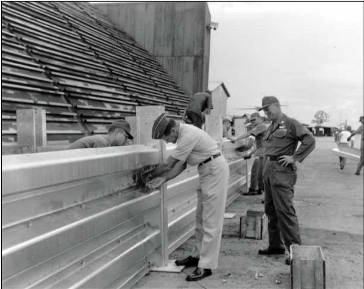
ADC Prime BEEF team gets top-level assistance in building aircraft revetments from Lt. Gen. Joseph H. Moore, Commander of 2d Air Division, as Lt. Col. Francis. H. Torr "supervises."
