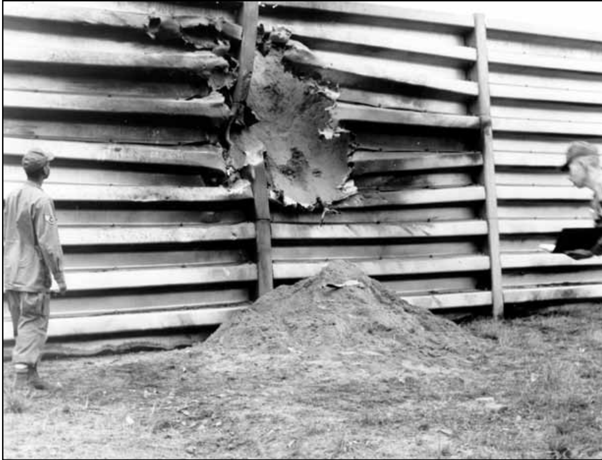
It worked! The revetment at Da Nang AB received a direct hit from a 122mm rocket during a Viet Cong attack on the base in January 1968.
