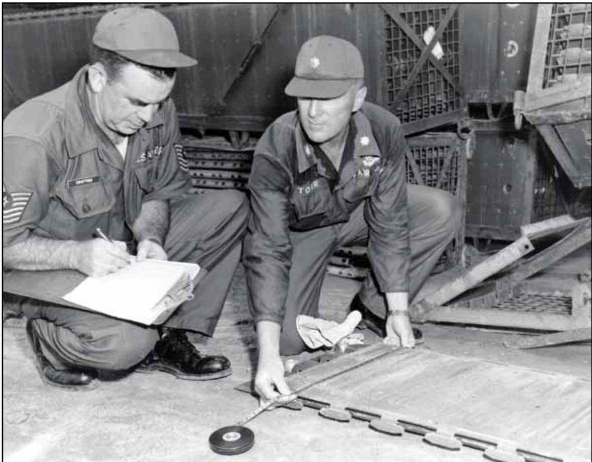
Lt. Col. Francis E. Torr (right) and MSgt Bruce F. Swafford, members of Prime BEEF Team #1, measure AM-2 matting for use in aircraft revetments at Tan Son Nhut AB, South Vietnam, August 1965.
