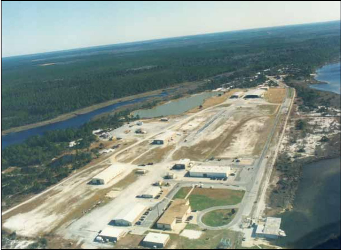
Aerial view of the 9700 Research and Testing Area, Tyndall AFB, Florida.
