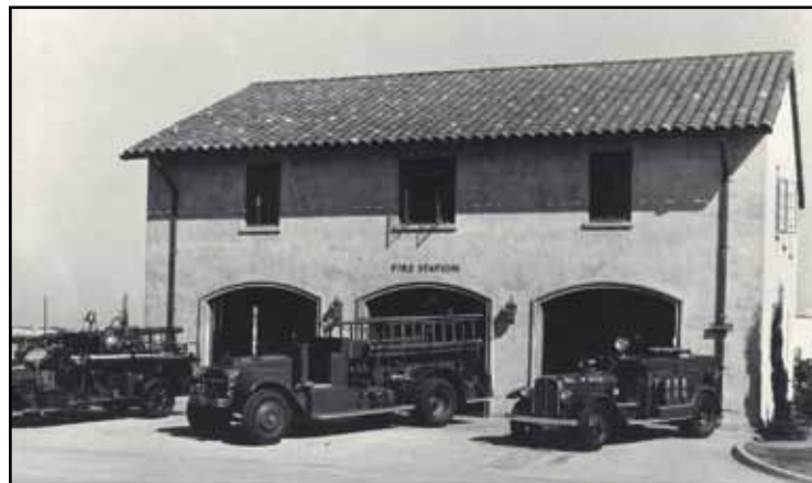
An early fire station at Randolph Field, Texas, built at a cost of $14,904 in 1930.
