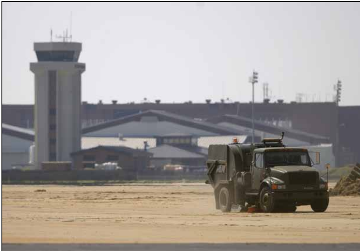
1st Civil Engineer Squadron sweepers clear the large amount of debris left by the receding flood waters on the Langley AFB parking areas following Hurricane Isabel.
