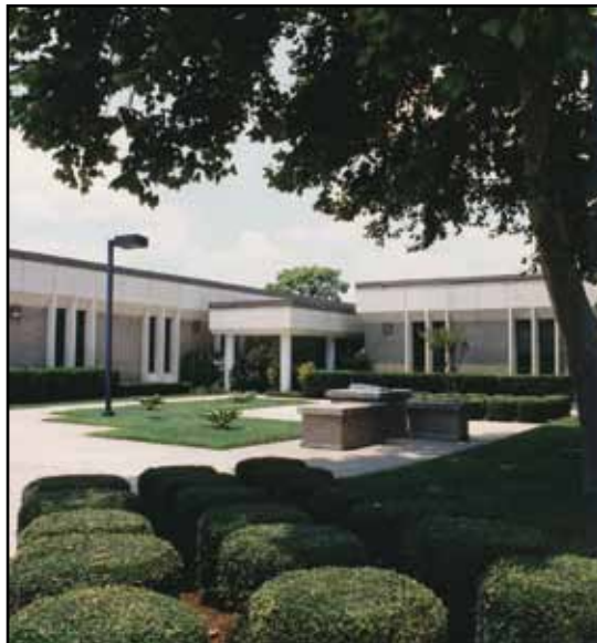
Exterior view of Building 1120, HQ Air Force Engineering and Services Center.
