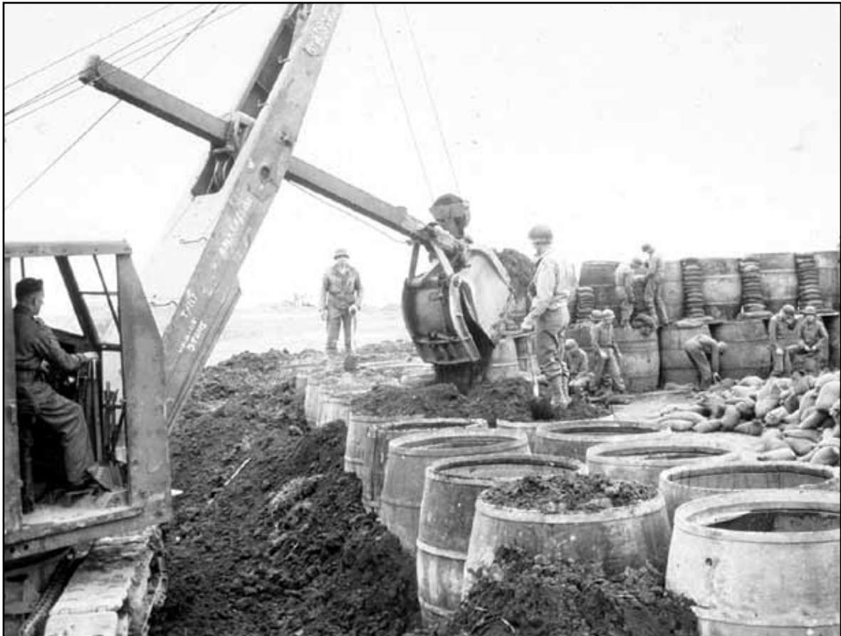
Aviation engineers used every available source of materials. Here they construct aircraft revetments using wooden wine barrels filled with dirt and sandbags near Anzio.
