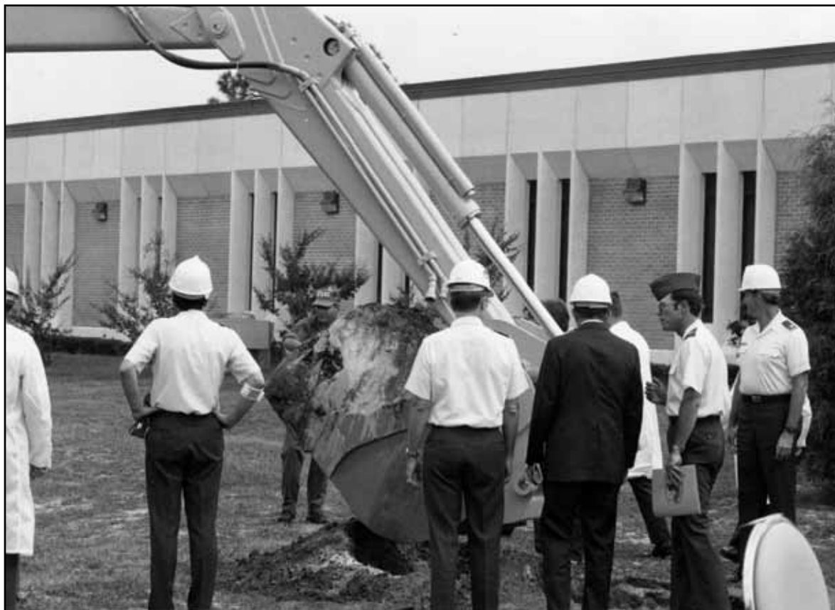
Groundbreaking for Building 1117, Engineering and Services Laboratory, Tyndall AFB, Florida.
