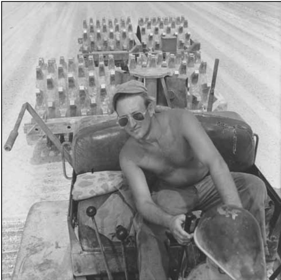
An aviation engineer pulls a sheepfoot roller during construction of an airfield on Saipan.
