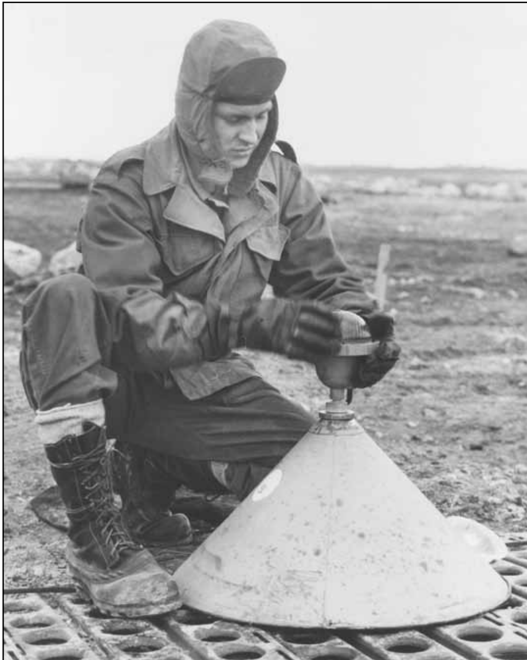
An Airman repairs a runway light at a Korean air base.
