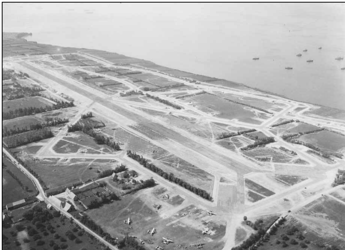
An airfield built by the 834th Engineer Aviation Battalion at St. Pierre Du Mont, France.
