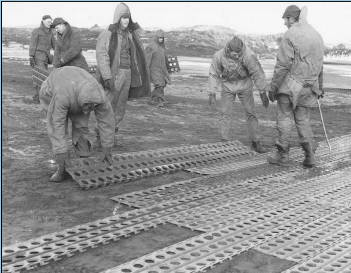
Aviation engineers in Alaska construct a runway using pierced steel plank.
