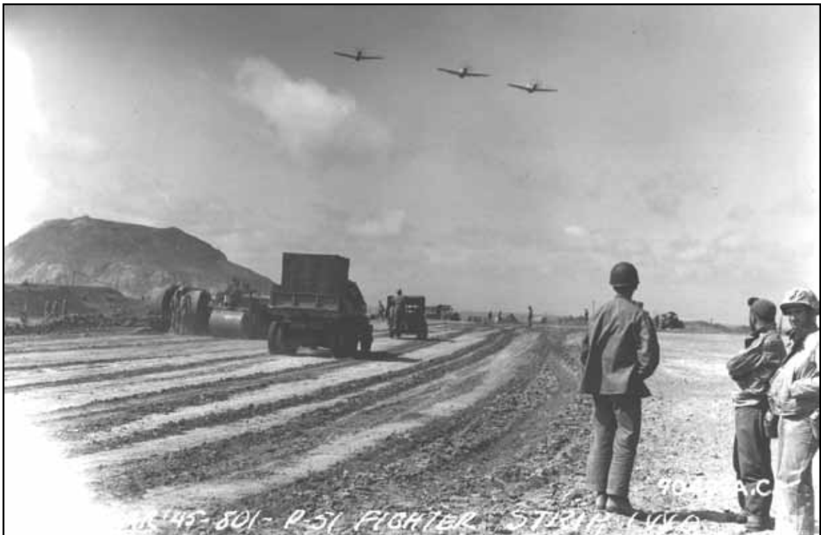
As P-51s fly overhead, engineers widen the south end of Number 1 airstrip on Iwo Jima, March 1945.
