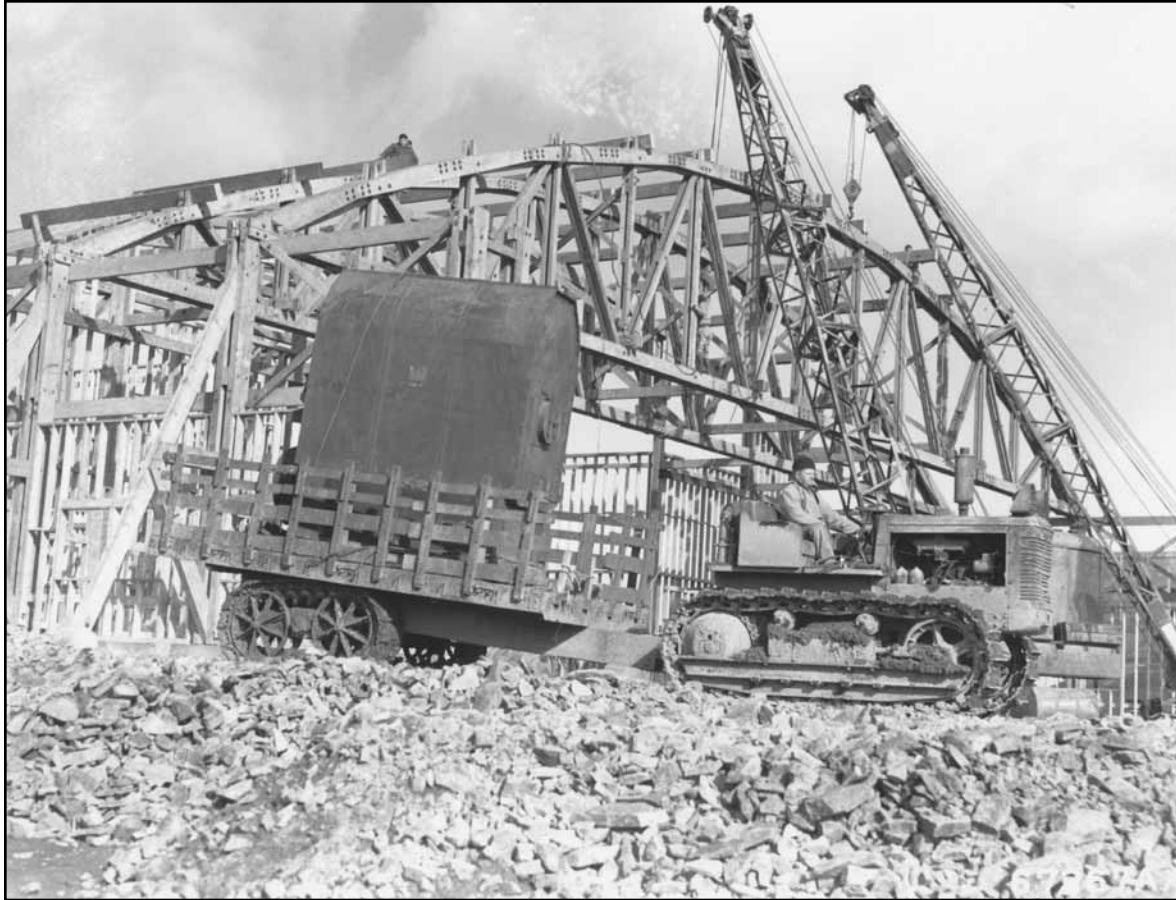
Buildings under construction at the southern tip of Amchitka, Alaska, 1943.
