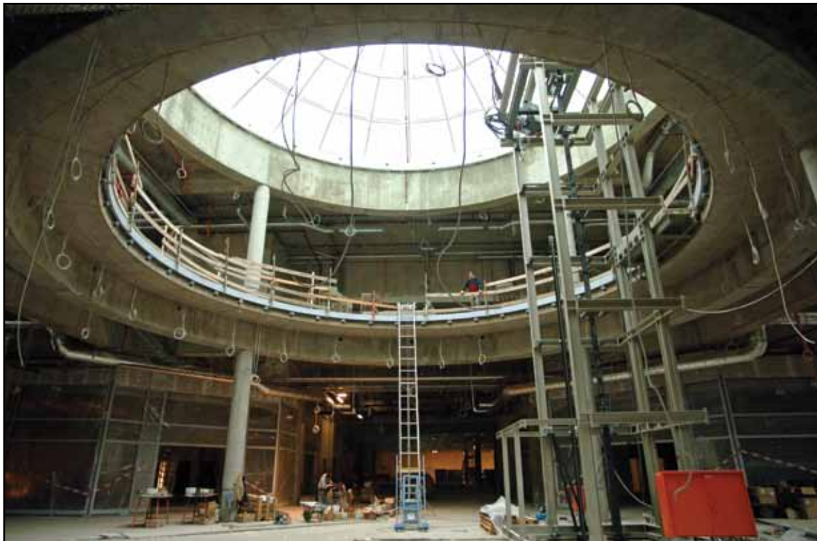
Construction of the Kaiserslautern Military Community Center at Ramstein AB, Germany.
