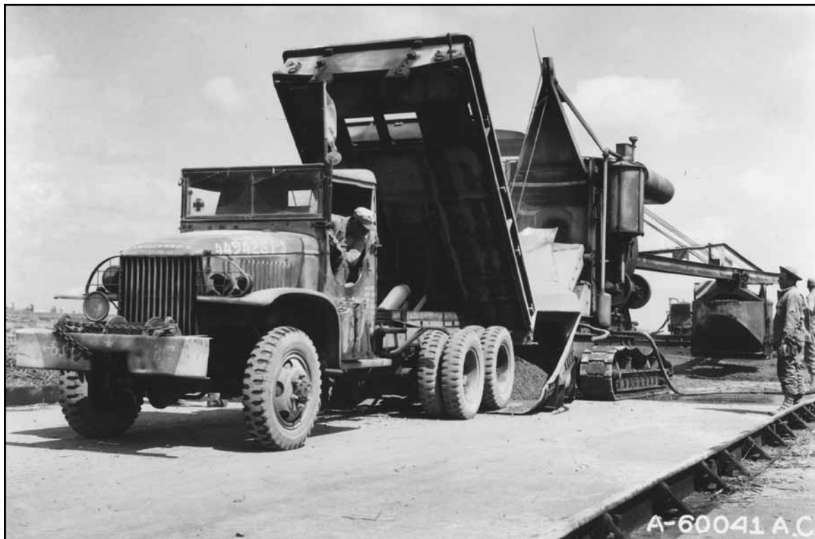
Members of the 831st Engineer Aviation Battalion at work in England.
