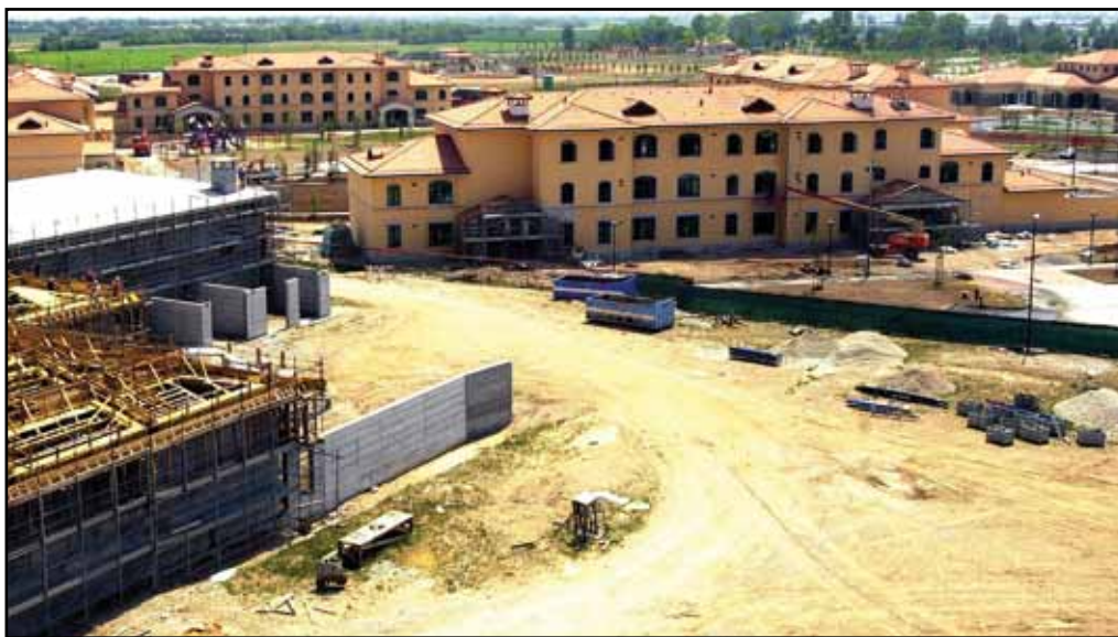
Part of Aviano Air Base’s $540 million construction on the Aviano 2000 Program.
