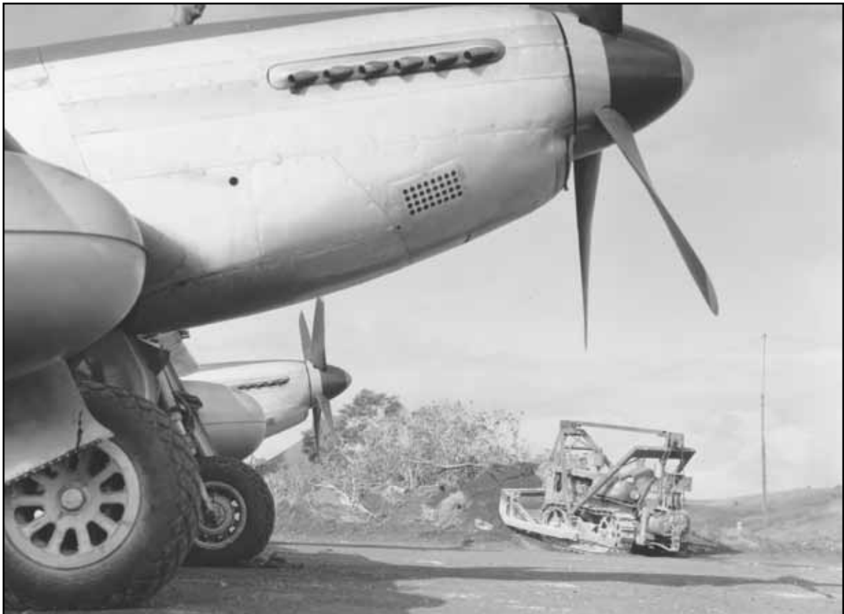
At East Field, Saipan, a seven-ton D-4 tractor clears the jungle to provide parking space for P-51s.
