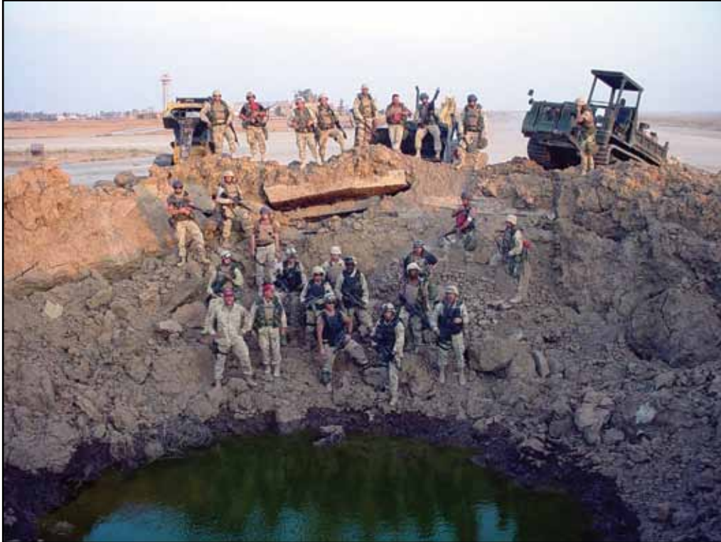
An Airborne RED HORSE team poses in the “Mother of all Craters” at Baghdad International Airport before beginning repairs. The crater was 135 feet wide and 40 feet deep and filled with water 15 feet deep.
