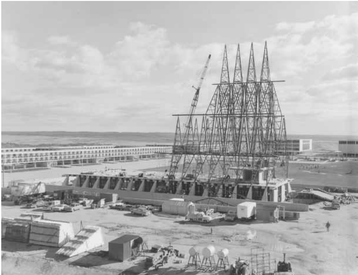
The U.S. Air Force Academy's iconic Chapel takes shape as the spires are set in place.
