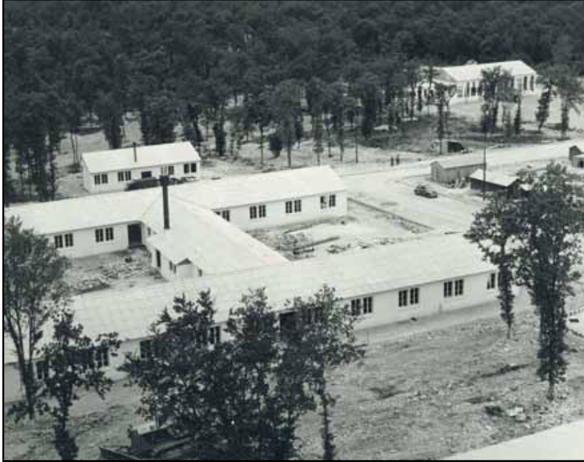
The Joint Construction Agency constructed a NATO ammunition depot in the Forest of Chizé near Niort, France, in 1947.
