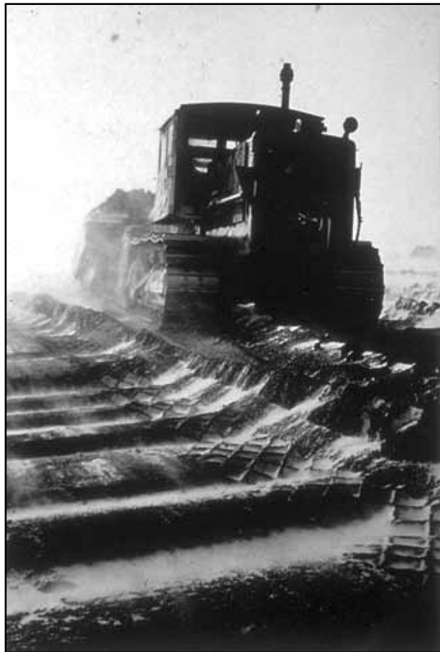
Construction at a Distant Early Warning site.
