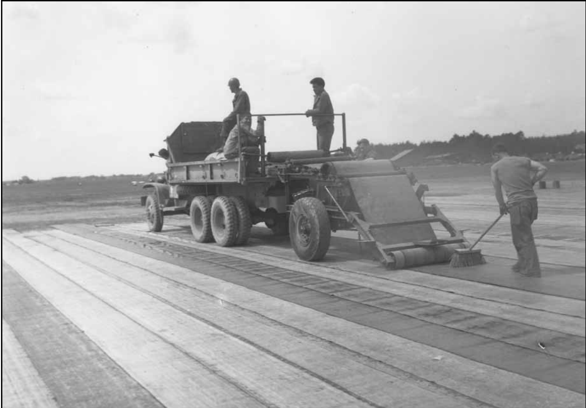
Members of the IX Engineer Command build an airfield using Hessian Matting in Normandy, France.
