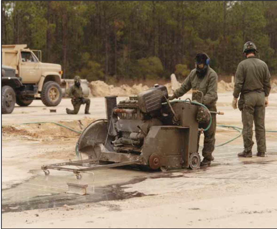
Civil engineers participate in rapid runway repair training at Eglin's Field 4.
