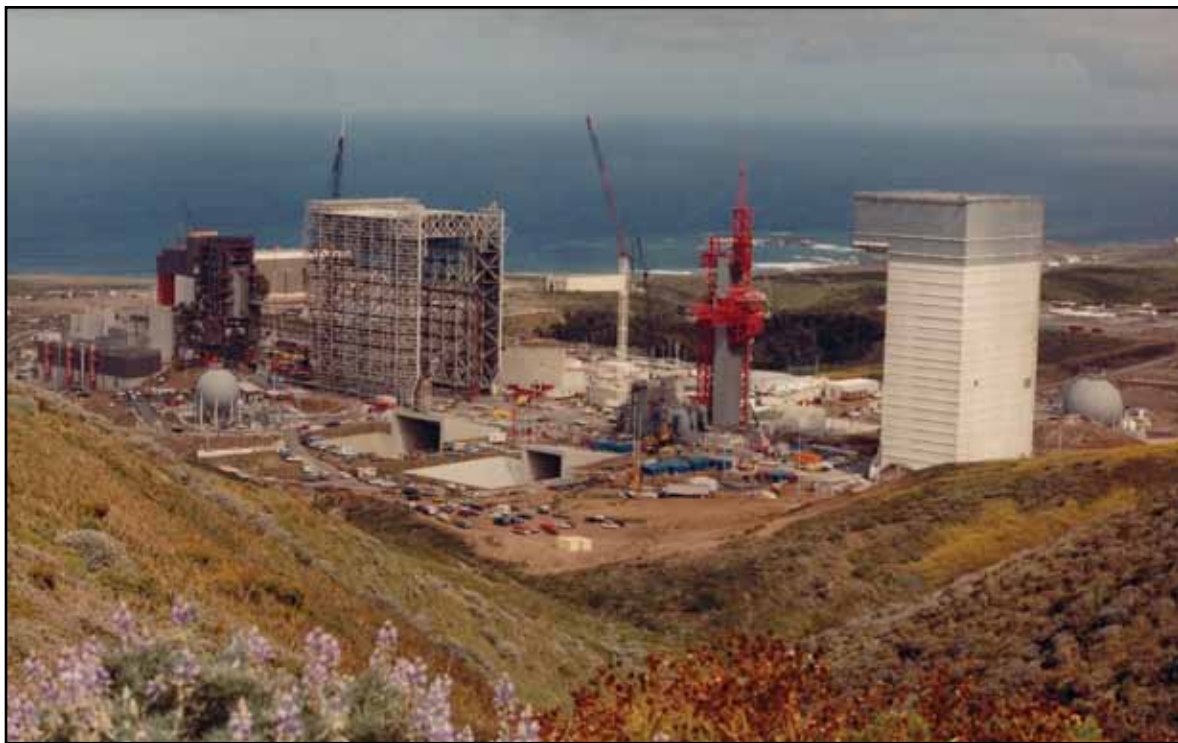
Space Launch Complex 6 at Vandenberg AFB, California.
